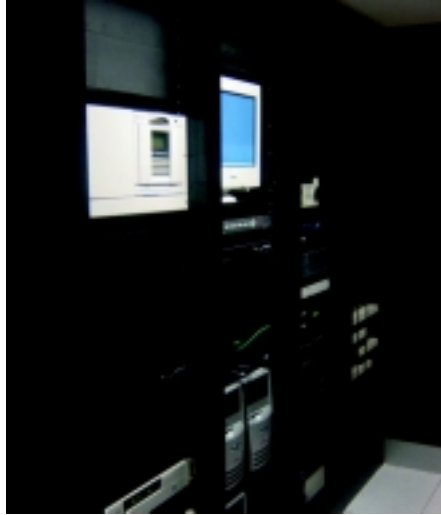
The moot court server rack.
